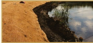
Soil Erosion Control
